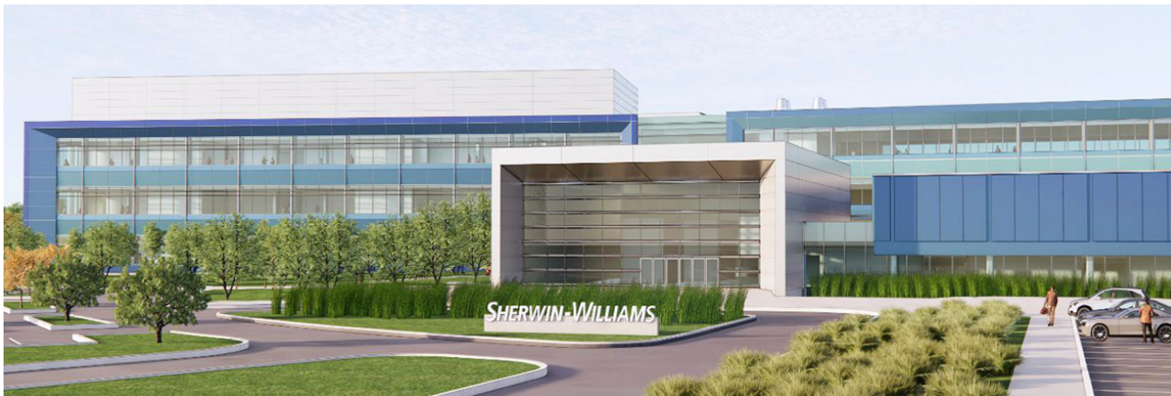
Sherwin-Williams expects to move into its new research and development center in Brecksville, Ohio, sometime in 2025. Chemists, engineers, technicians and support teams will work in the center, part of company's Building Our Future project.
